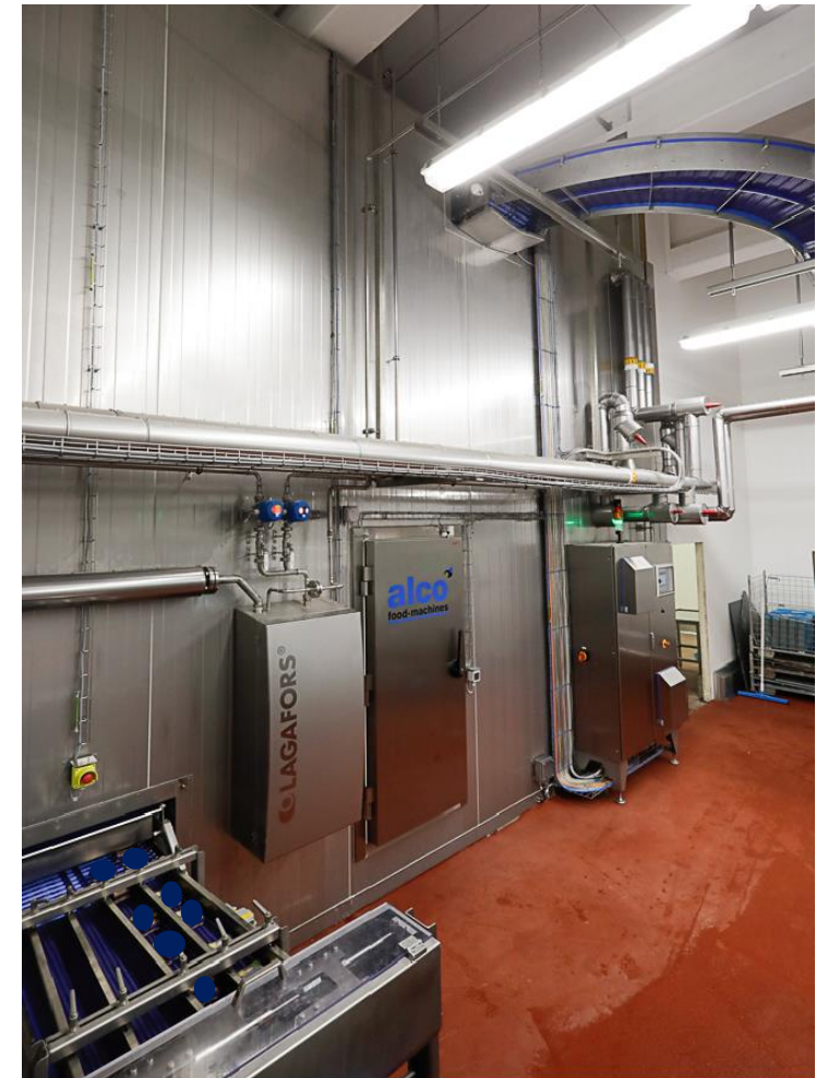
Finished Spiral Freezer ASK at a customer's site
